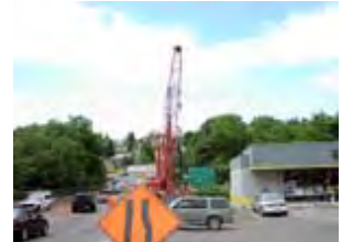
Marine View Drive Bridge
