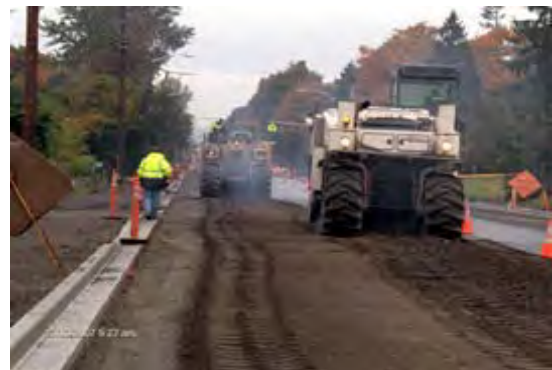
16th Avenue S. Paving Preparation (10.16.07)
