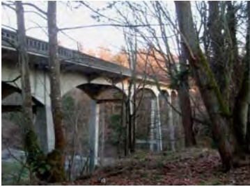
Saltwater State Park Bridge
