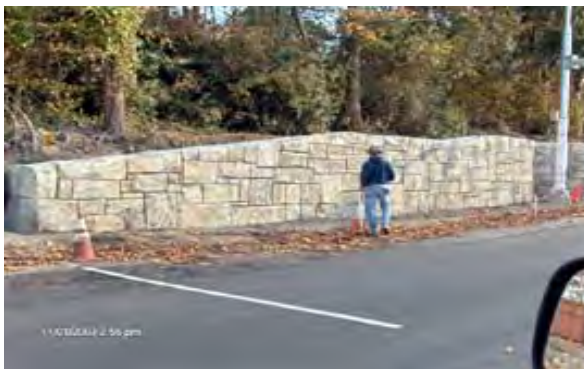
Retaining Wall near S. 260th St. (11.01.07)
