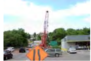
Marine View Drive Bridge
