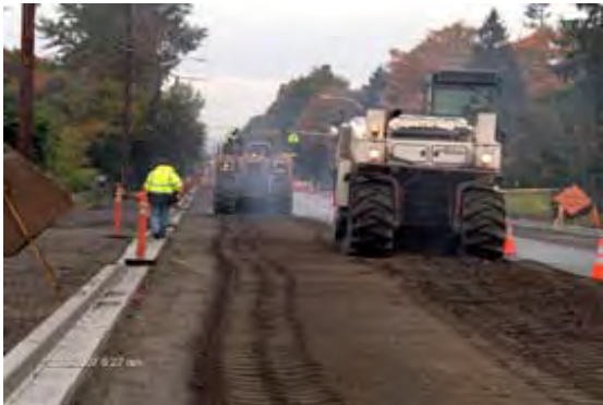
16th Avenue S. Paving Preparation (10.16.07)
