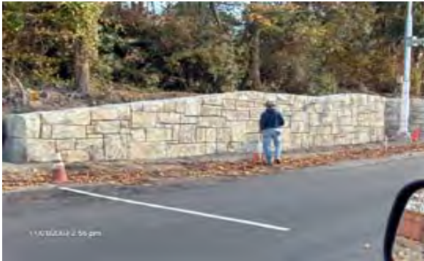
Retaining Wall near S. 260th St. (11.01.07)
